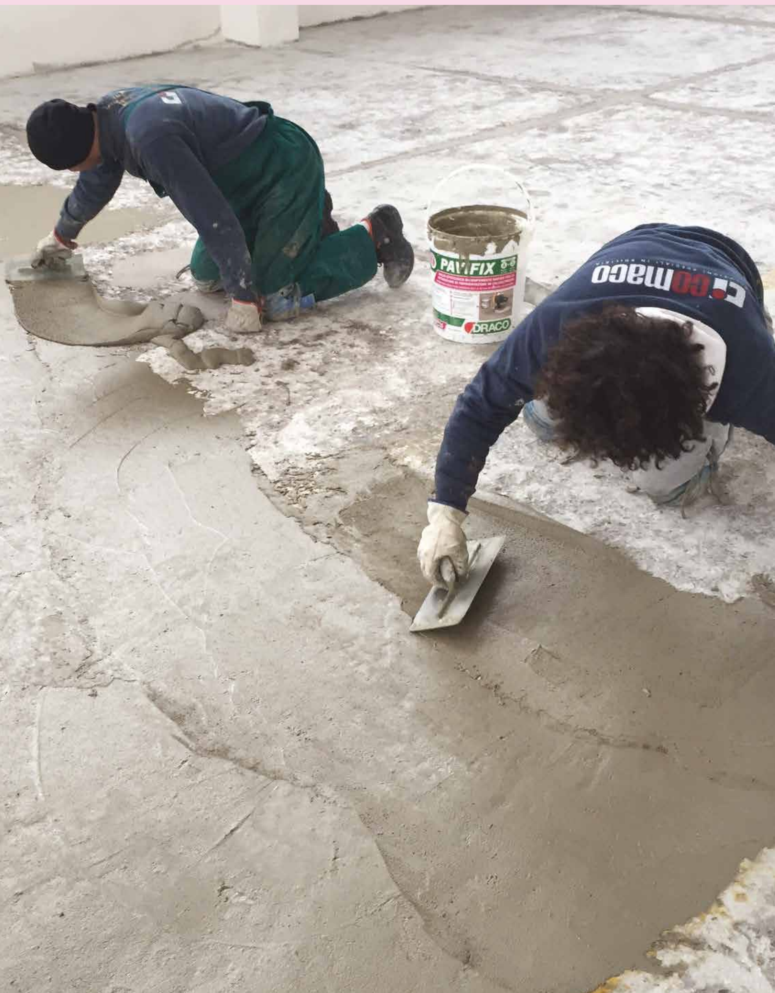
MAAR Group factory - Isola d'Elba, Livorno, Italy Smoothing and structural repair of flooring with cement-based resin EPOMALT FAST 100.
