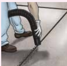
Cut and clean the joint.
