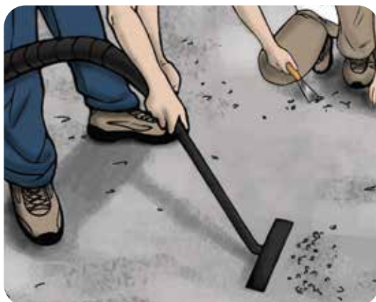
• Thoroughly clean the substrate.
