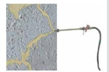
At the pre-set gel time the monomer solution gels, thus creating a polymer lattice that incorporates the molecules of infiltration water and also triggers a water-repelling action against water present.
