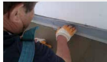
HIDROIZOLACIJA BALKONA I ESTRIHA SUSTAVOM MAGIFLEX TERRAZZO
