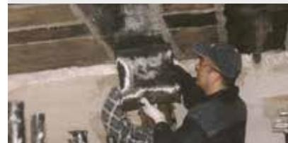
TKANINE I LAMELE OD UGLJIKOVIH VLAKANA ZA UČVRŠĆIVANJE I KONSTRUKCIJSKU ARMATURU
