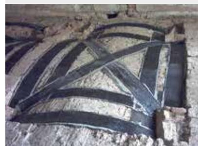
TKANINE I LAMELE OD UGLJIKOVIH VLAKANA ZA UČVRŠĆIVANJE I KONSTRUKCIJSKU ARMATURU
