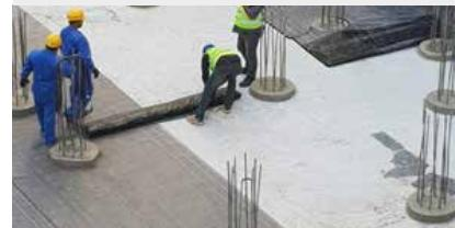
HIDROIZOLACIJA BETONSKIH TEMELJA I KONSTRUKCIJA, UKLJUČUJUĆI PODZEMNE, TEHNOLOGIJOM NA BAZI BENTONITA
