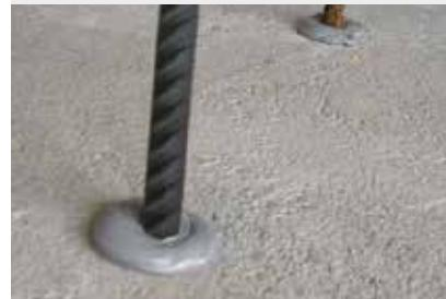
TIKSOTROPNA EPOKSIDNA LJEPILA ZA KONSTRUKCIJSKO SIDRENJE I LIJEPLJENJE
