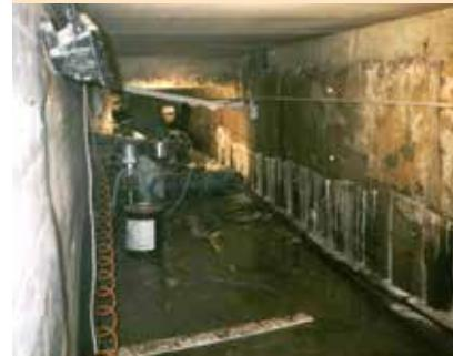
POLIURETANSKE HIDROEKSPANZIVNE SMOLE ZA UČVRŠĆUJUĆE INJEKTIRANJE I HIDROIZOLACIJU
