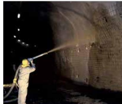
DODACI ZA UBRZAVANJE VEZIVANJA BETONA I PRSKANIH MORTOVA (SPRITZ-BETON)
