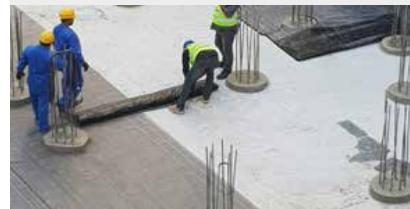
HIDROIZOLACIJA BETONSKIH TEMELJA I KONSTRUKCIJA, UKLJUČUJUĆI PODZEMNE, TEHNOLOGIJOM NA BAZI BENTONITA
