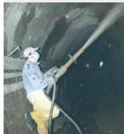
DODACI ZA UBRZAVANJE VEZIVANJA BETONA I PRSKANIH MORTOVA (SPRITZ-BETON)
