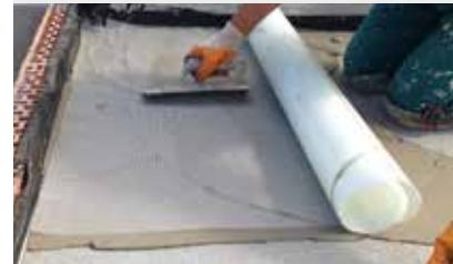
HIDROIZOLACIJA BALKONA I ESTRIHA SUSTAVOM MAGIFLEX TERRAZZO
