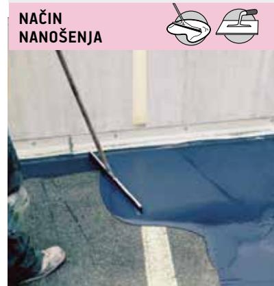
SMOLE ZA POPRAVKE I OBLOGE ASFALTA I BITUMENSKIH KOLNIKA
