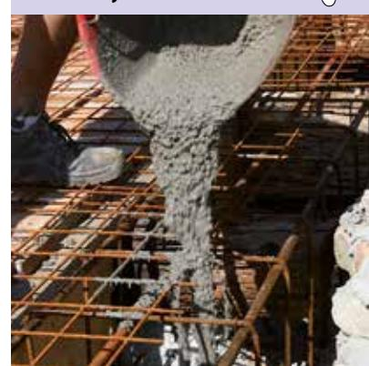
CEMENTNE INJEKCIJSKE SMJESE KOJE SE MOGU LIJEVATI ZA RESTAURACIJU I POVEĆANJE DEBLJINE BETONSKIH KONSTRUKCIJA
