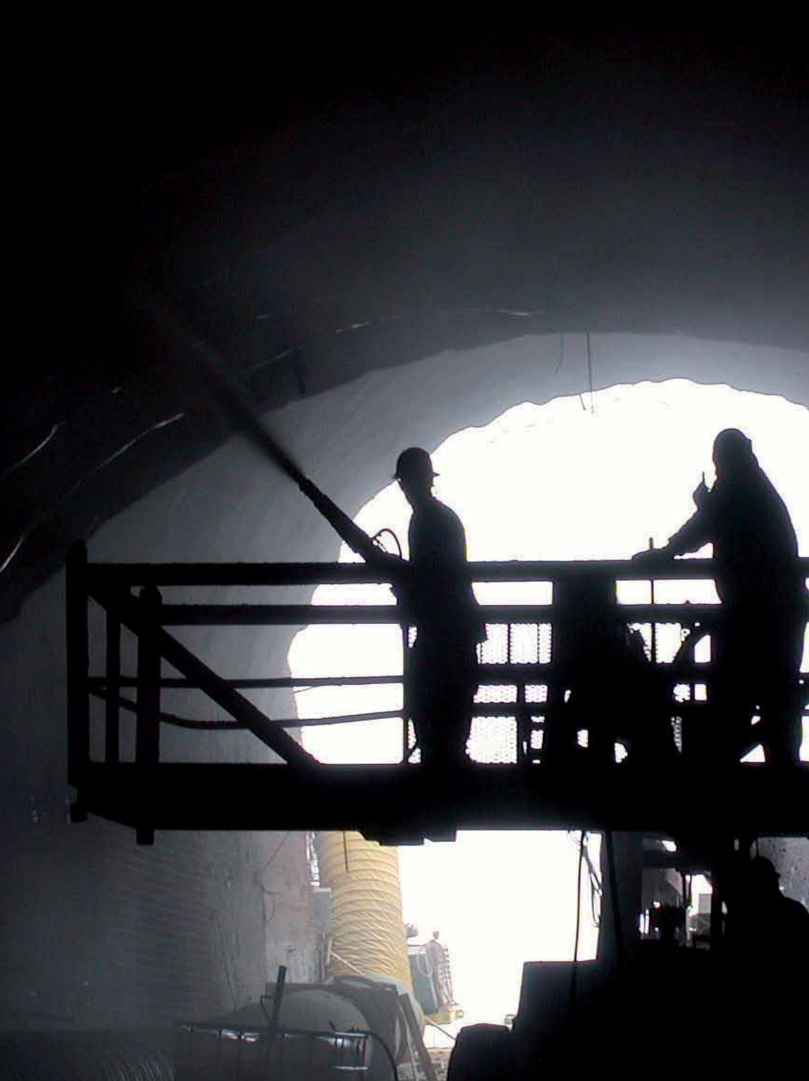
Monte Giglio tunnel, Calusco d'Adda, Bergamo Tunnel shotcrete prepared with FIBERFLEX S and DRANITE AF
