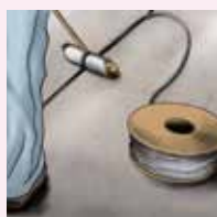
■ Positioning the DRAFIL cord to form a support.
