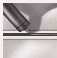
■ Application of the flexible polyurethane sealant, EPOJOINT .
