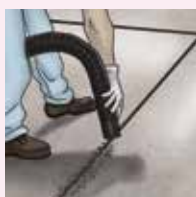
■ Cutting and cleaning of joint.
