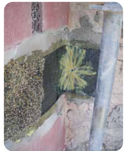
3. OPENING AND FASTENING OF THE THREAD
