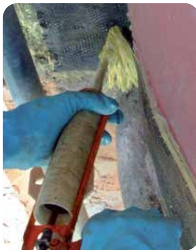
2. FILLING AND IMPREGNATION WITH EPOXY RESIN
